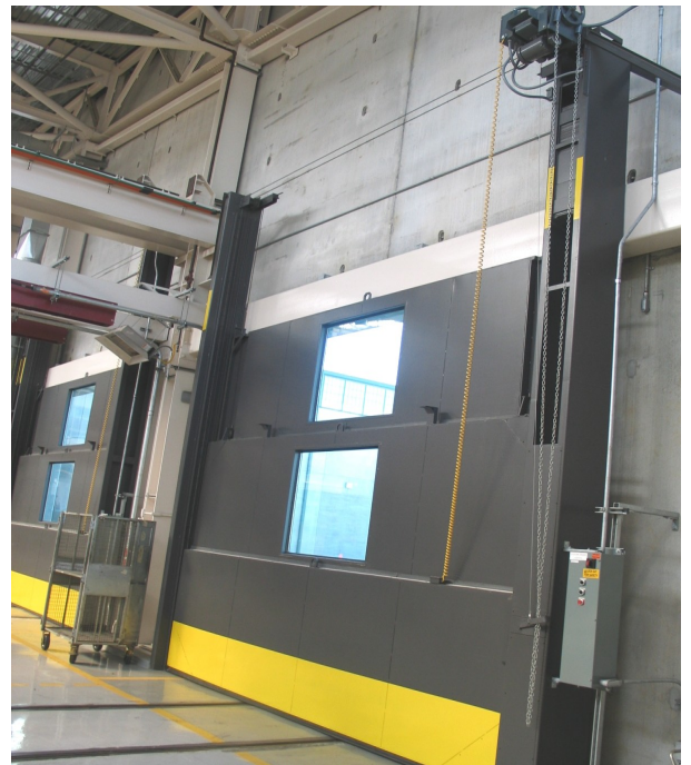
1 PSI Three Panel Vertical Lifting Fueling Door for Metro Transit System Garage
