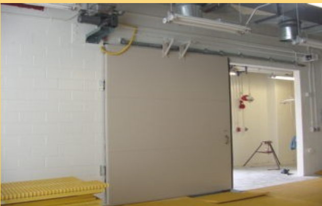
Blast and Fire Rated Sliding Door with Explosion Proof Operator for Chemical Storage
