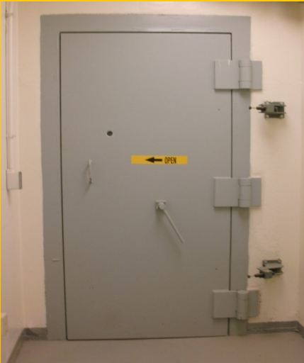
270 PSI Blast Door With Air Tight, Chemical Resistant Seals and Sight Hole
