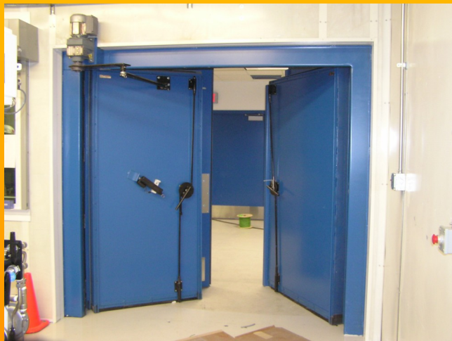
STC 60, Blast and Fragment Resistant Door with Power Operators and Latches
