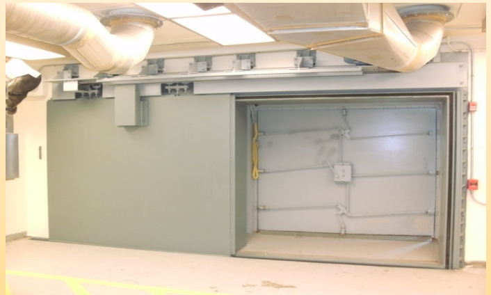
344 PSI Sliding Blast Door - Fragmentation Pneumatically Sealed- Gas Tight Under Full Gas and Shock Phase Load
