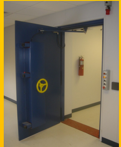
80 PSI Power Operated Designed for 100% Rebound
