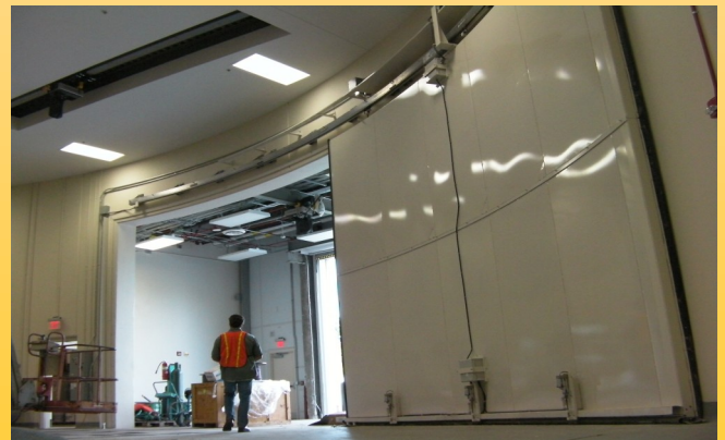
Curved Pressure Resistant Door STC 50 Acoustical rating
