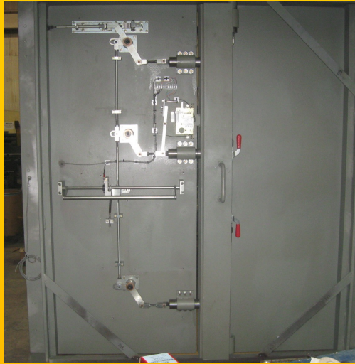
50 PSI, 3 hr Fire Rated Blast Door with Custom Panic Hardware
